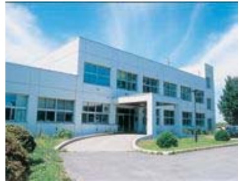
管理棟 Administration Building, Fujisaki Farm ①
