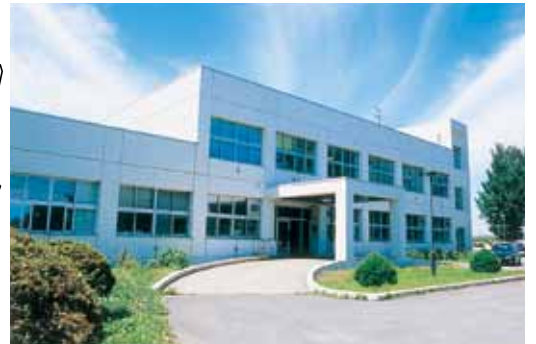
管理棟 Administration Building, Fujisaki Farm ①
